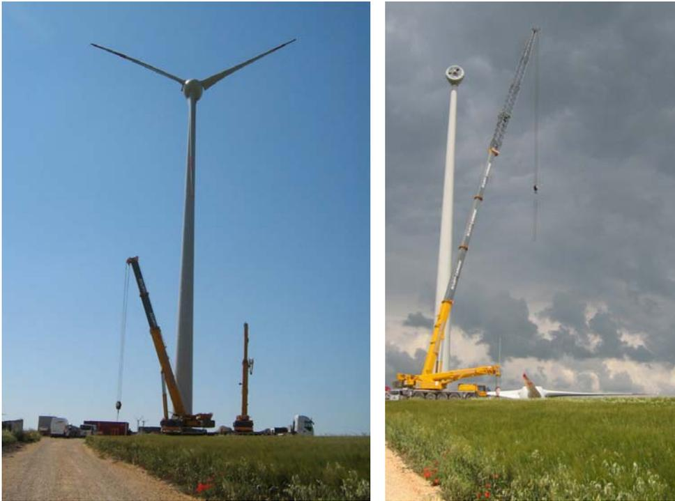
**Figura 2:** rimozione eliche e mozzo
