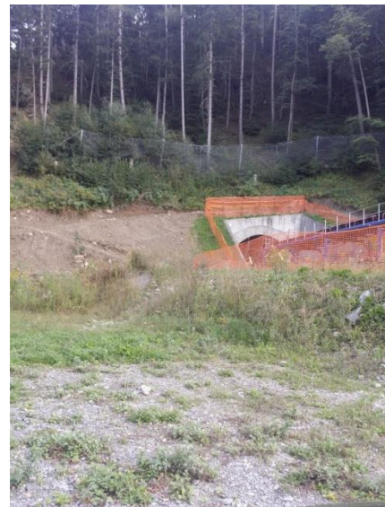
Portal Aicha-Hinterrigger Portale Aica-Hinterrigger
