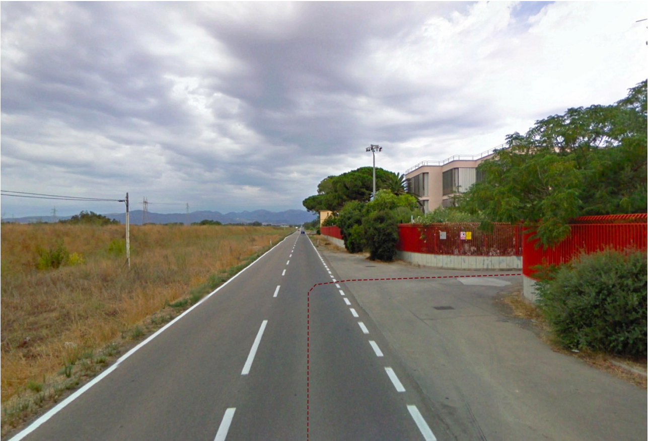
Vista 18_Ingresso SSE 380 kW Villasor
