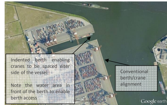
Figure 6-13 Indented berth at Amsterdam Container Terminal, Image from Google Earth Pro
