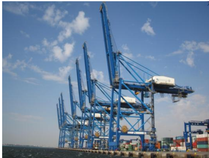
Figure 6-6 Typical Standard Ship to Shore Crane serving mainline vessel
