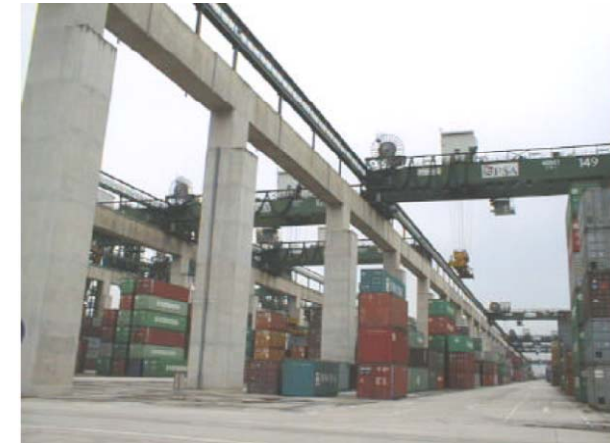
Figure 6-12 Automated overhead bridge cranes at Pasir Panjang Container Terminal Singapore (note these do not have a barge crane end and only serve the yard)
