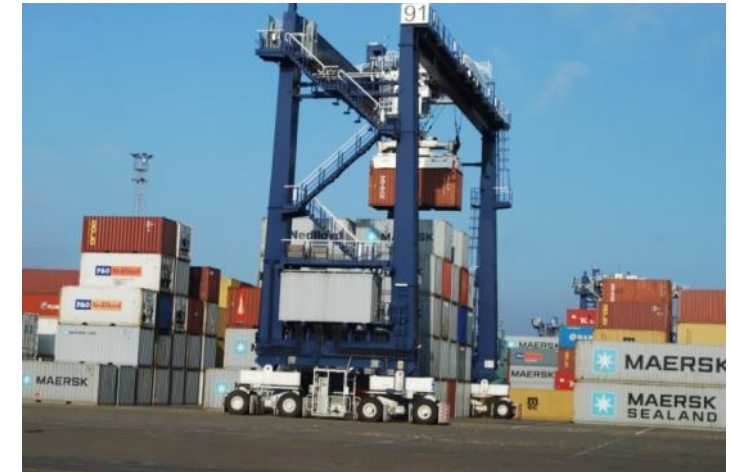
Figure 6-7 Typical rubber tyre gantry crane serving a stack
