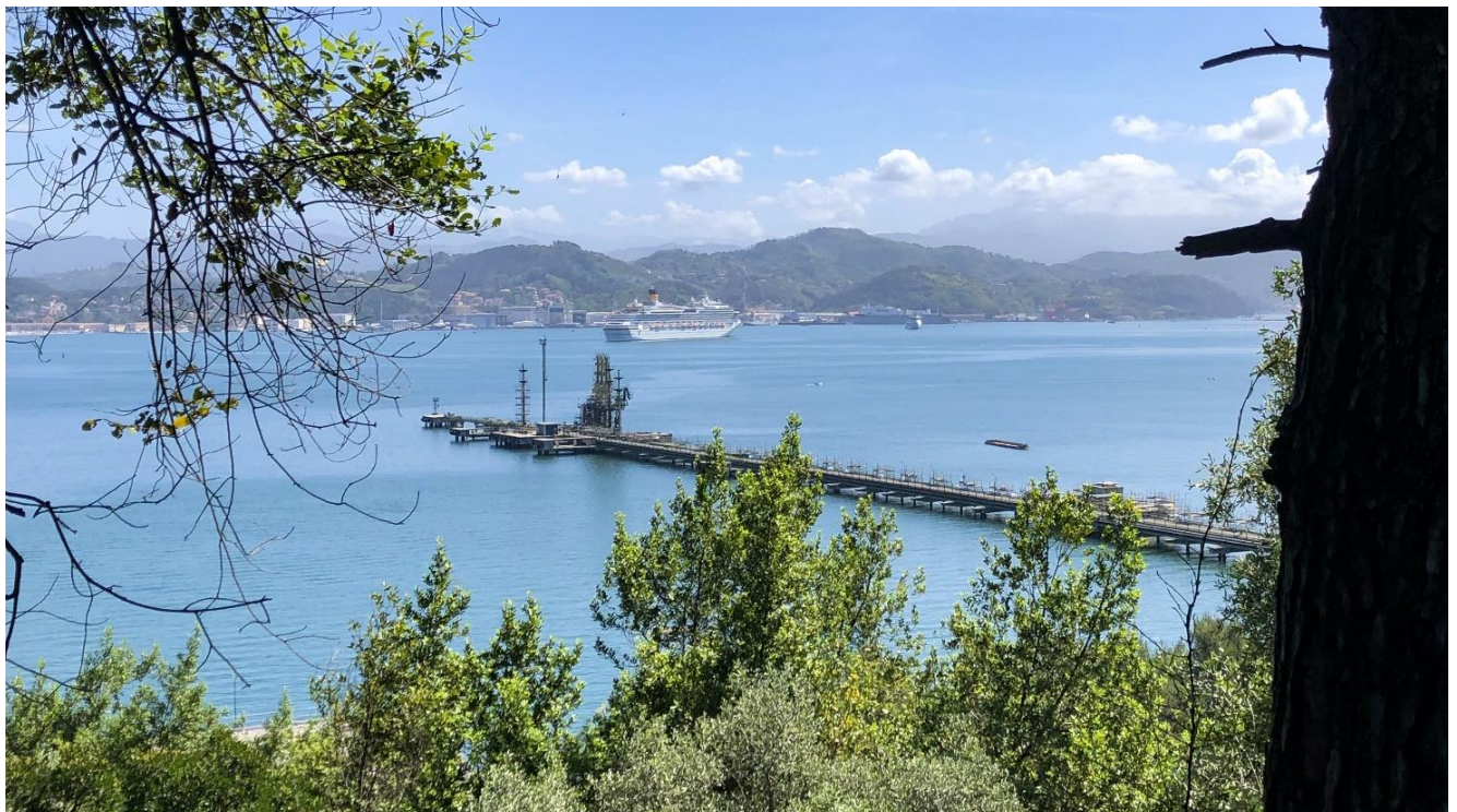
Figura 35: PV2 - Post operam
