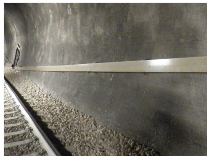
Rivestimento in spritz beton/gunite
