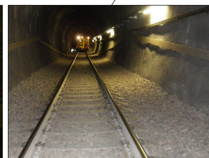
Rivestimento in spritz beton/gunite
