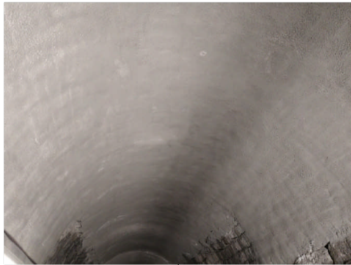
Rivestimento in spritz beton/gunite
