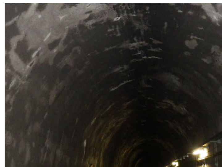
Rivestimento in spritz beton/gunite
