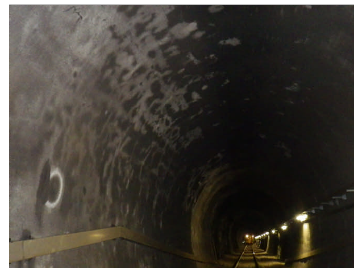
Rivestimento in spritz beton/gunite
