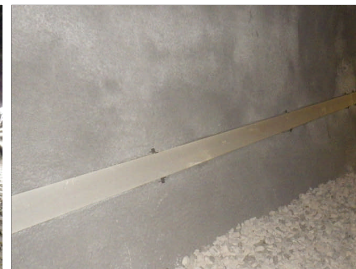
Rivestimento in spritz beton/gunite
