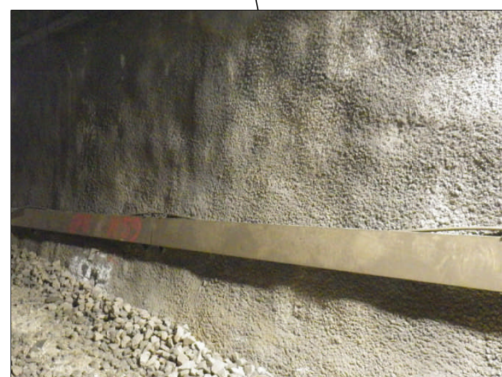
Rivestimento in spritz beton/gunite
