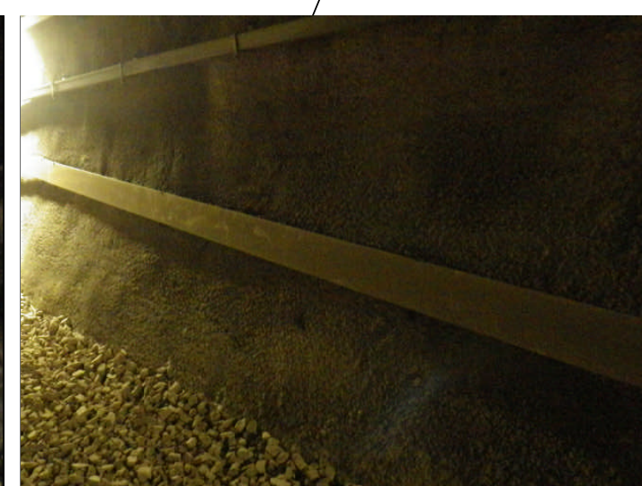
Rivestimento in spritz beton/gunite
