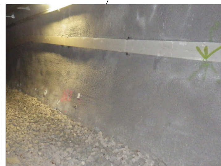
Rivestimento in spritz beton/gunite
