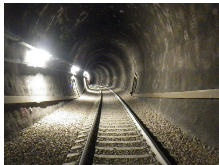
Rivestimento in spritz beton/gunite
