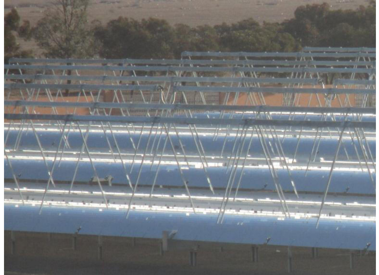
Morocco – FLT - Power generation
