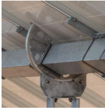
iTracker 1-axis PV tracker
