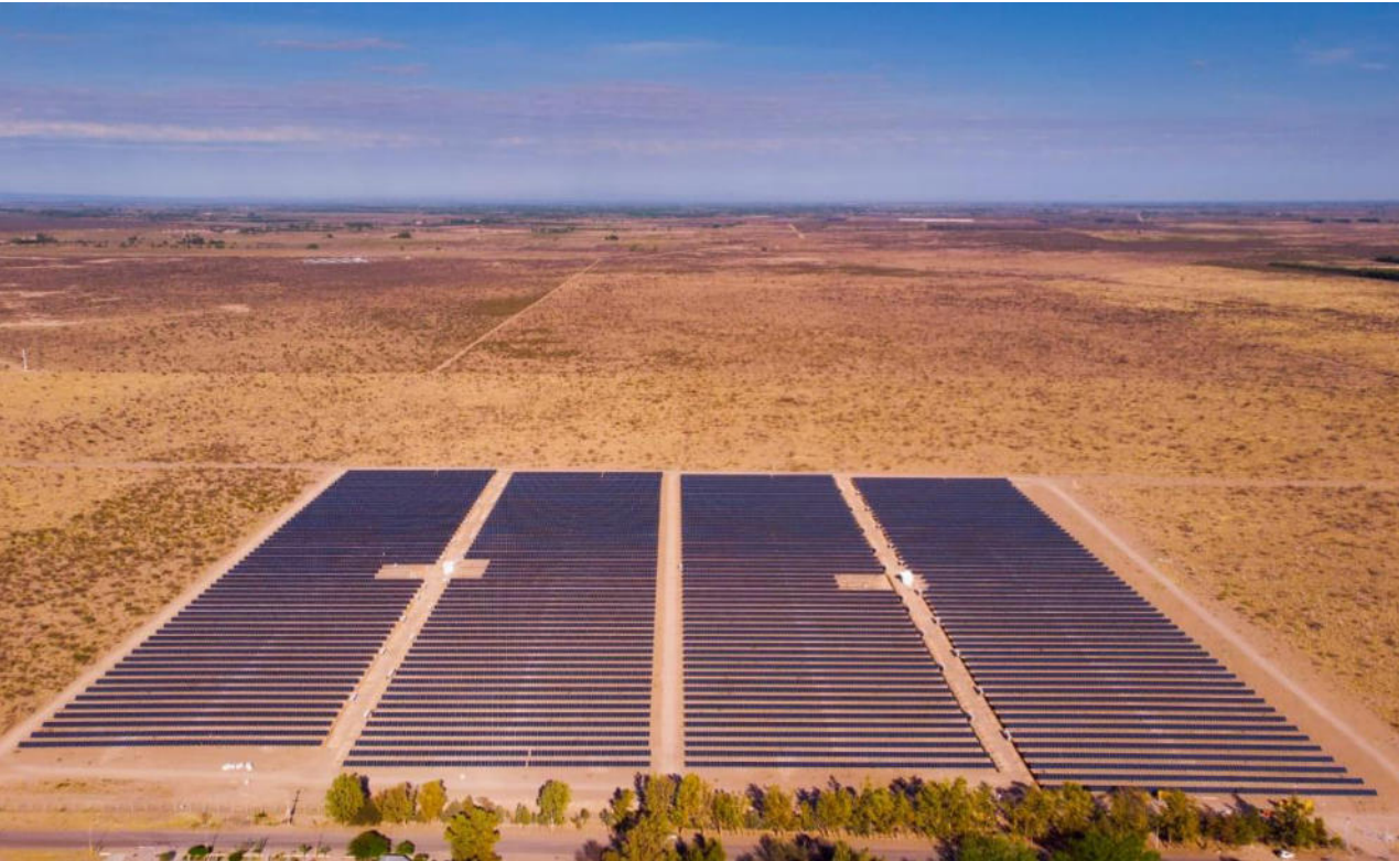
Argentina – 8 MWp, PV trackers
