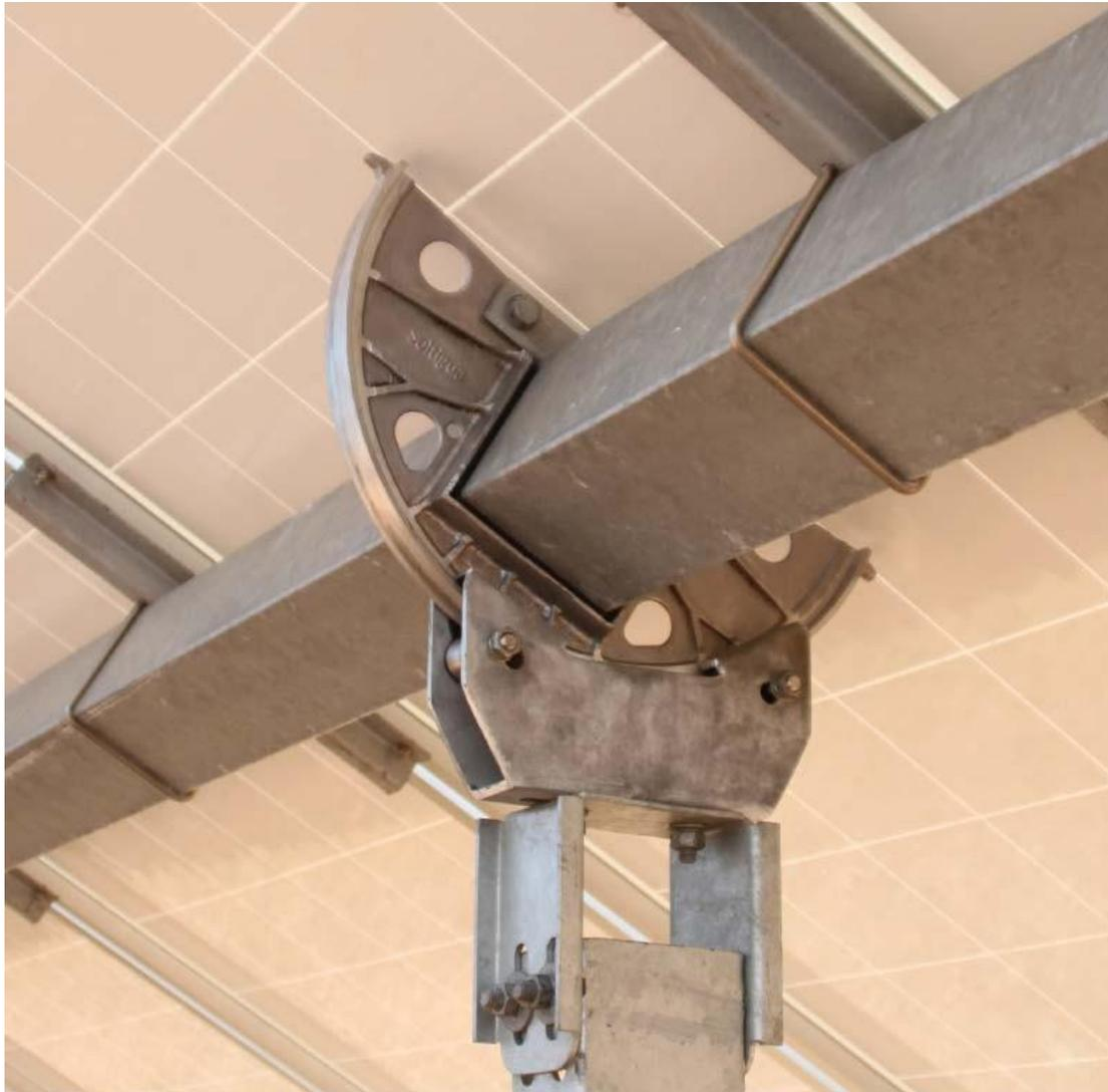
FIGURA 6: SCHEMA NODO TRAVE CONTINUA / COLONNA
