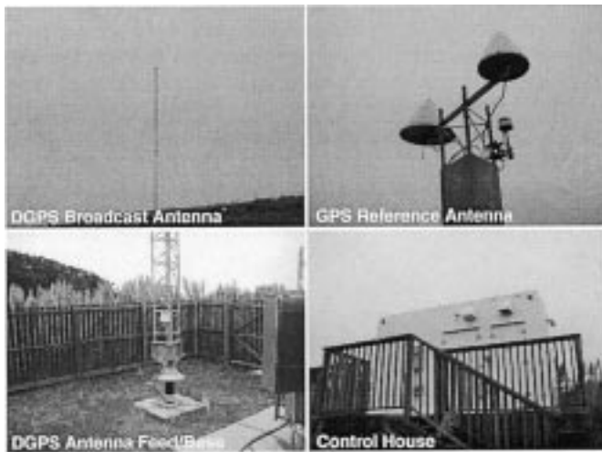
Fig. 3. NDGPS 287 kHz station at Pigeon Point, CA.
