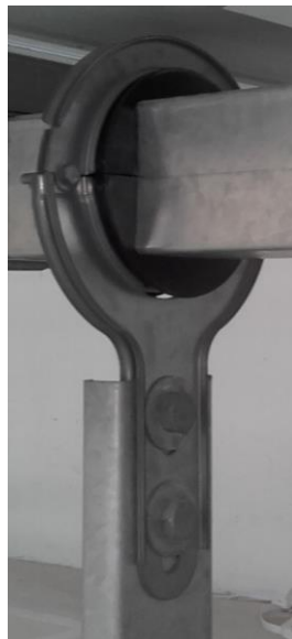
Figure 6. Joint between rotation beam and post
