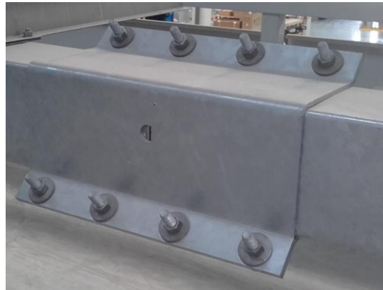
Figure 5. Joint between rotation beams
