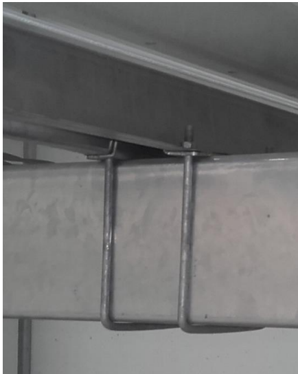
Figure 7. Joint between Panel rail and rotation beam
