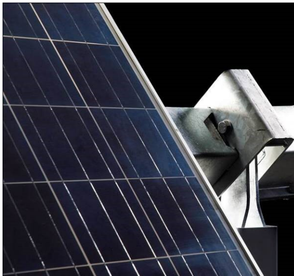
Intermediate Post-Head Detail
