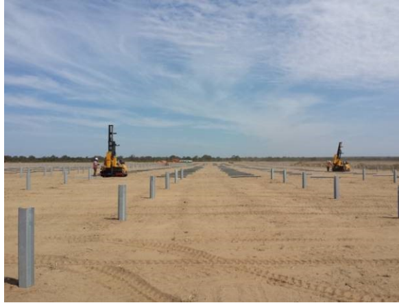
Driving omega piles phase
