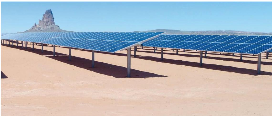
*Figura 3-3 - Tipico tracker configurazione portrait (fonte: <https://soltec.com/single-axis-solar-tracker/>)*
