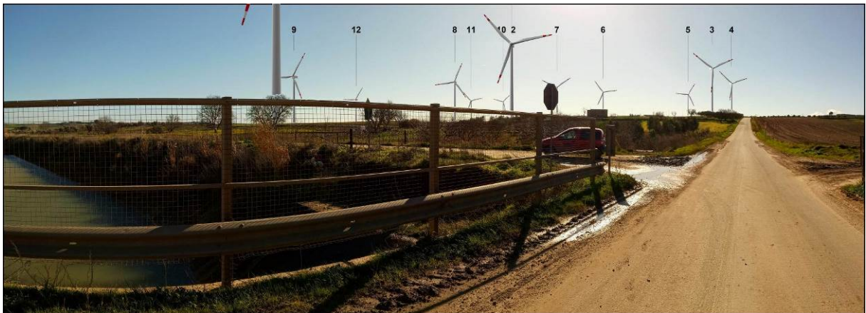
Vista V1_1 post operam
