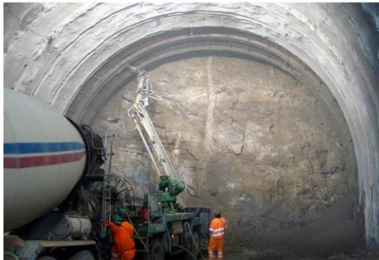
**Figura 25: Messa in opera spritz beton sulle centine.**
