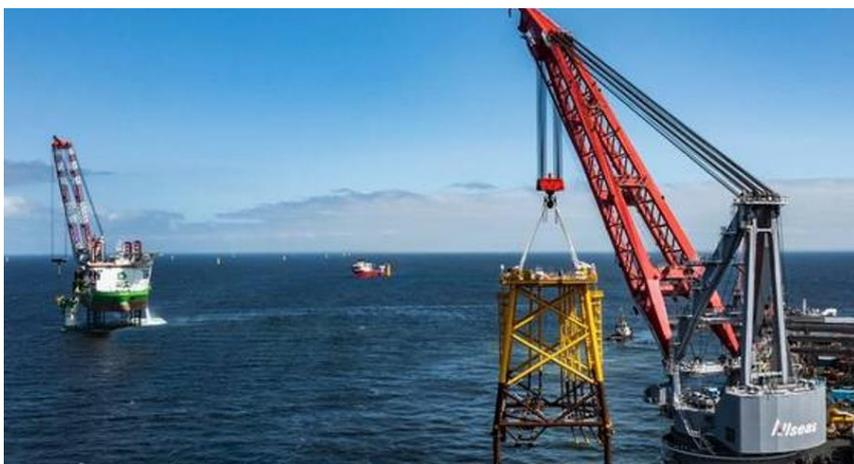
Figura 3.18 \_ Installazione: Jacket lifting and lowering
