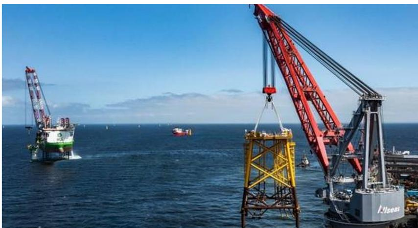
Figura 6.18 \_ Installazione: Jacket lifting and lowering
