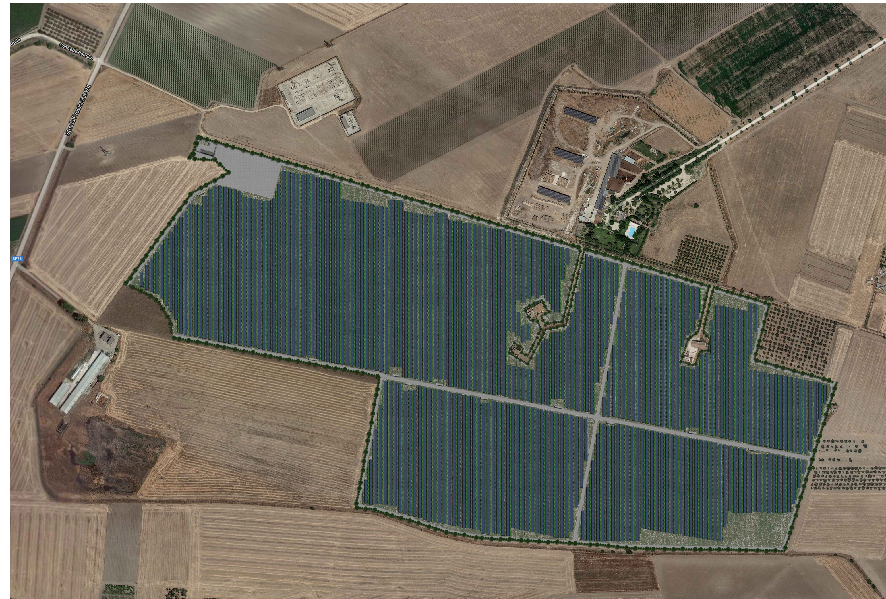
ORTOFOTO POST OPERAM
