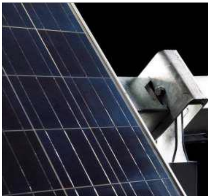
Intermediate Post-Head Detail
