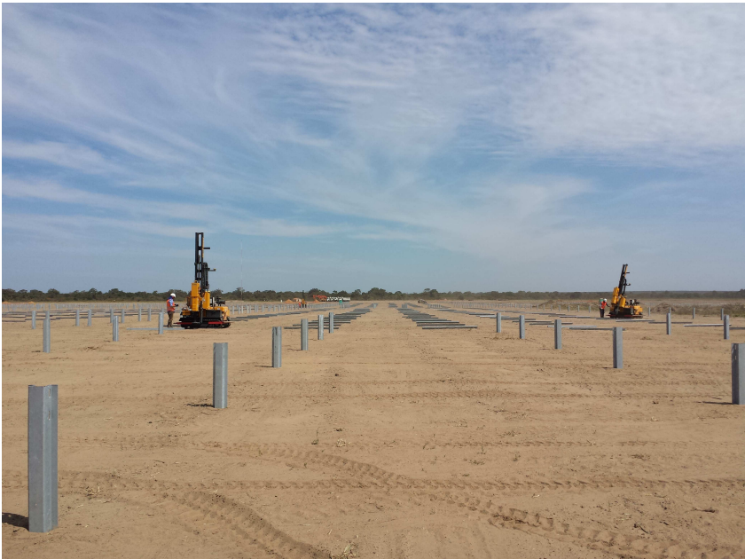
Figure 4: Driving omega piles phase
