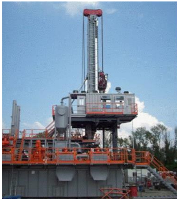
Figura 5.1: Impianto Drillmec HH-200MM
