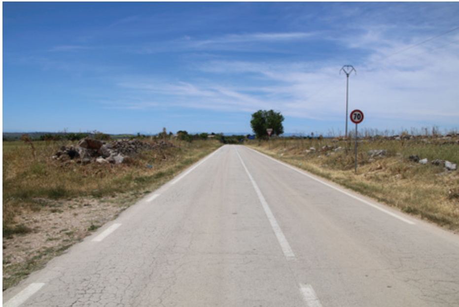
IMG_6659_Mass_IESCE_SP 160_verso AREA 5_6_7.JPG
