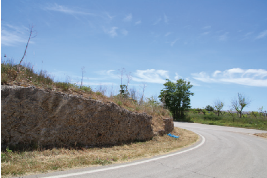
IMG_6658_Mass_IESCE_SP 160_verso AREA 5_6_7.JPG
