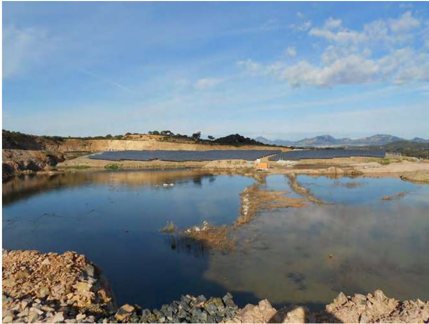
Fig. 13. 1 MW p photovoltaic system at Azza Ruja, in a brownfield (former mine). In order to create suitable condition for reconstituting a damaged ecosystem, the system has been designed with the consultancy of landscape designers by CIPNES (an administrative body devoted to the planning of industrial areas). Image courtesy of CIPNES.
