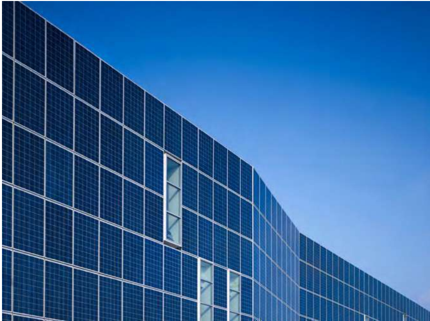
Fig. 4. Façade with opaque standard photovoltaic modules, allowing for building's energy self-sufficiency, and therefore characterized by a dense pattern, with associate high surface use energy intensity. Green Dot Animo Leadership High School, Inglewood, California, 2013. Design: Brooks+Scarpa Architects. Image courtesy of Larry Scarpa.
