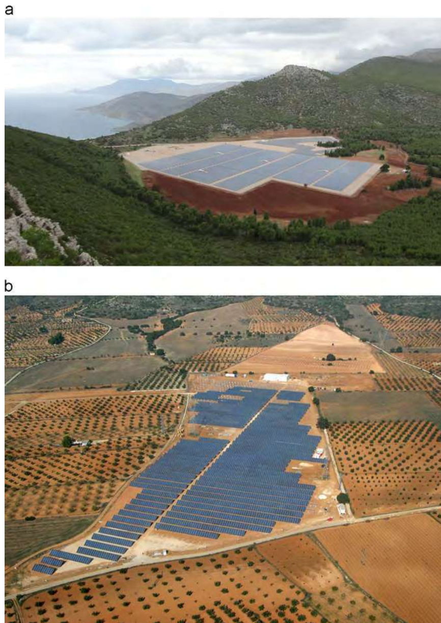
Fig. 2. (a) 1.5 MW p photovoltaic array, Vathihori-Psatha, Attiki (GR). (b) A section of a 20 MW p photovoltaic array, Beneixama (ES). Large photovoltaic arrays cause visible land and landscape transformations, due to their size; the impacts they generate depend on the features of the landscape in which they are placed. The "standard" visual result is a dense area covered by photovoltaic modules, organized in parallel stripes East–West oriented.
