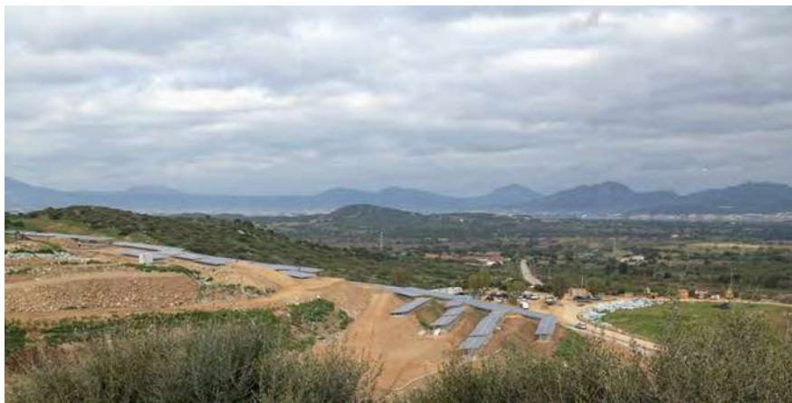
Fig. 14. 1 MW p photovoltaic system at landfill Spiritu Santo. In order to create suitable condition for reconstituting a damaged ecosystem, the system has been designed with the consultancy of landscape designers by CIPNES (an administrative body devoted to the planning of industrial areas). Image courtesy of CIPNES.
