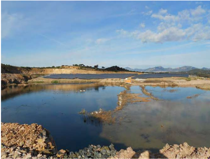
Fig. 13. 1 MW p photovoltaic system at Azza Ruja, in a brownfield (former mine). In order to create suitable condition for reconstituting a damaged ecosystem, the system has been designed with the consultancy of landscape designers by CIPNES (an administrative body devoted to the planning of industrial areas). Image courtesy of CIPNES.
