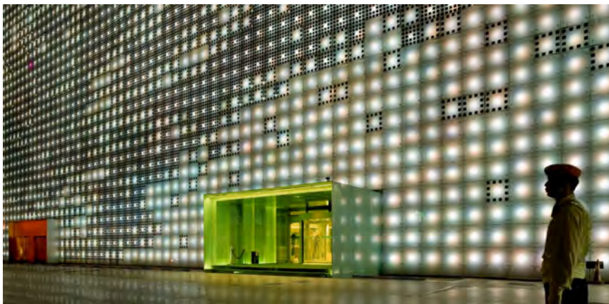
Fig. 5. Façade with semi-transparent glass-glass photovoltaic modules, allowing for a “natural,” random effect, and characterized by a porous pattern, and associated low surface use energy intensity. Green Pix, Beijing, China, 2008. Design: Simone Giostra. Image courtesy of Simone Giostra.
