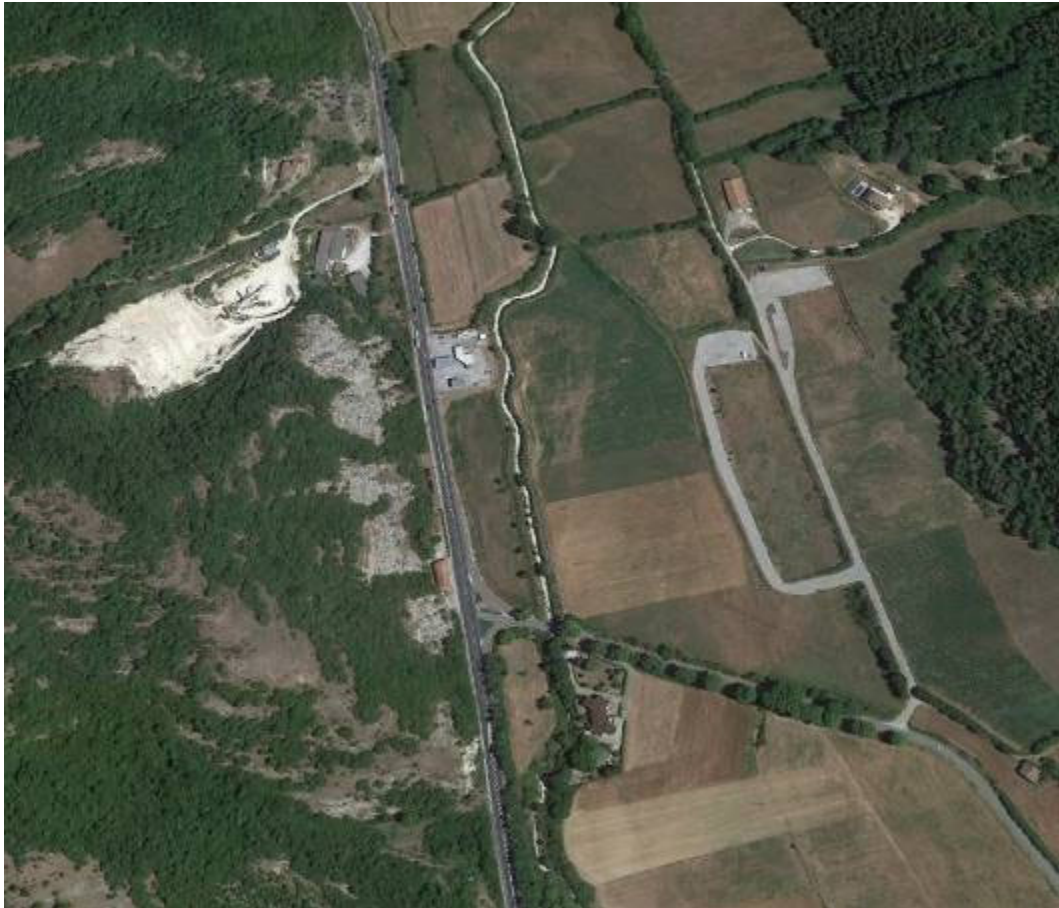
Figura 7.19 – Area cantiere SGR2
