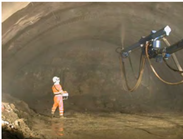
Figura 2.30 – Posa spritz-beton
