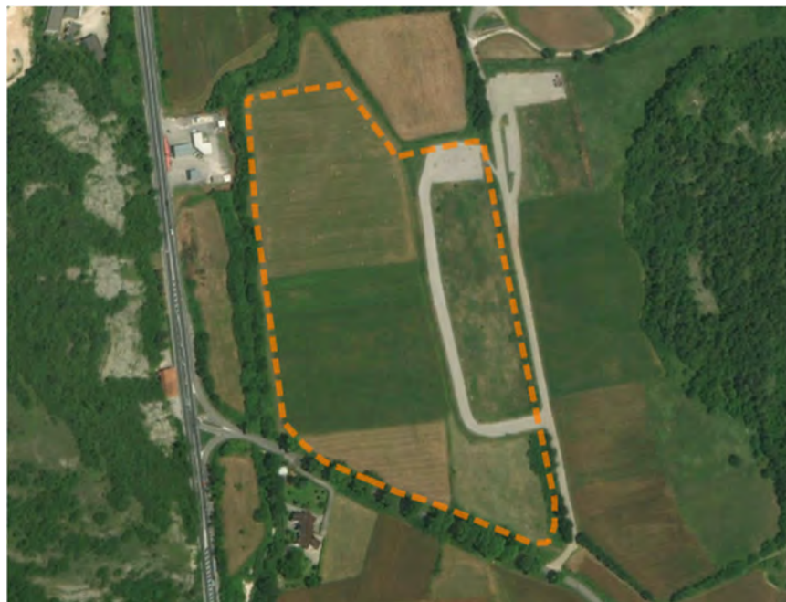
Figura 2.23 – Area cantiere SGR2
