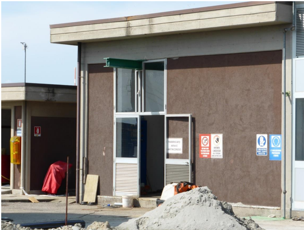
Figure 15: Building Containing Firewater Pumps
