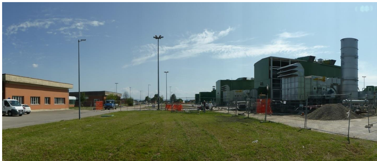
Figure 14: Location of the Compressor Enclosures in Relation to the Admin/Control Buildings
