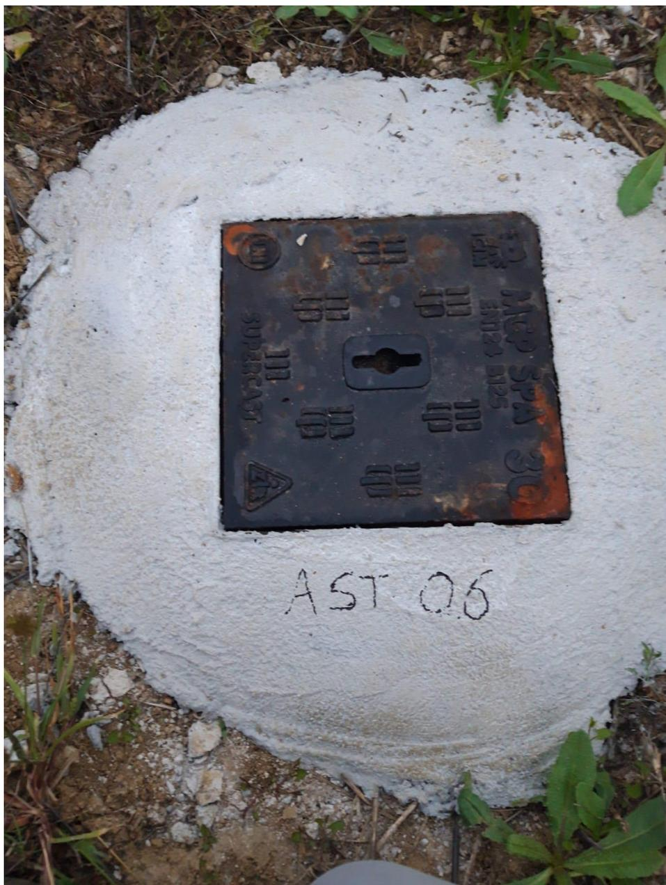
**FIGURA N. 18 - Piezometro AST\_06**
