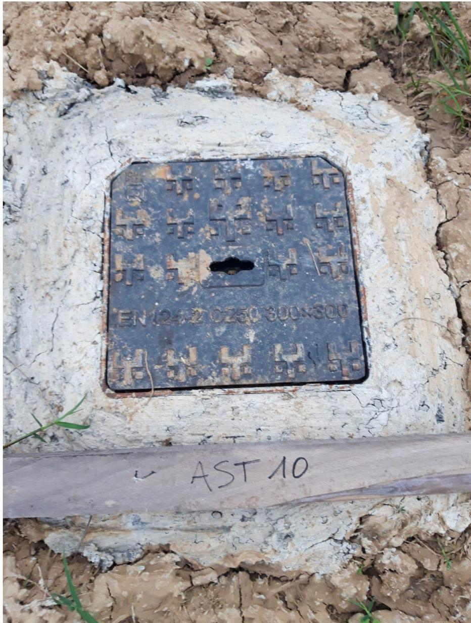
**FIGURA N. 22 - Piezometro AST\_10**
