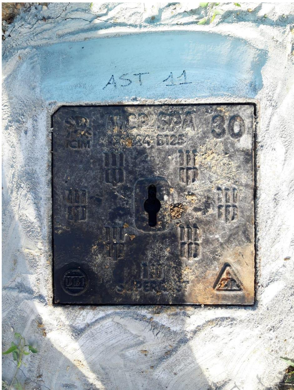
**FIGURA N. 23 - Piezometro AST\_11**
