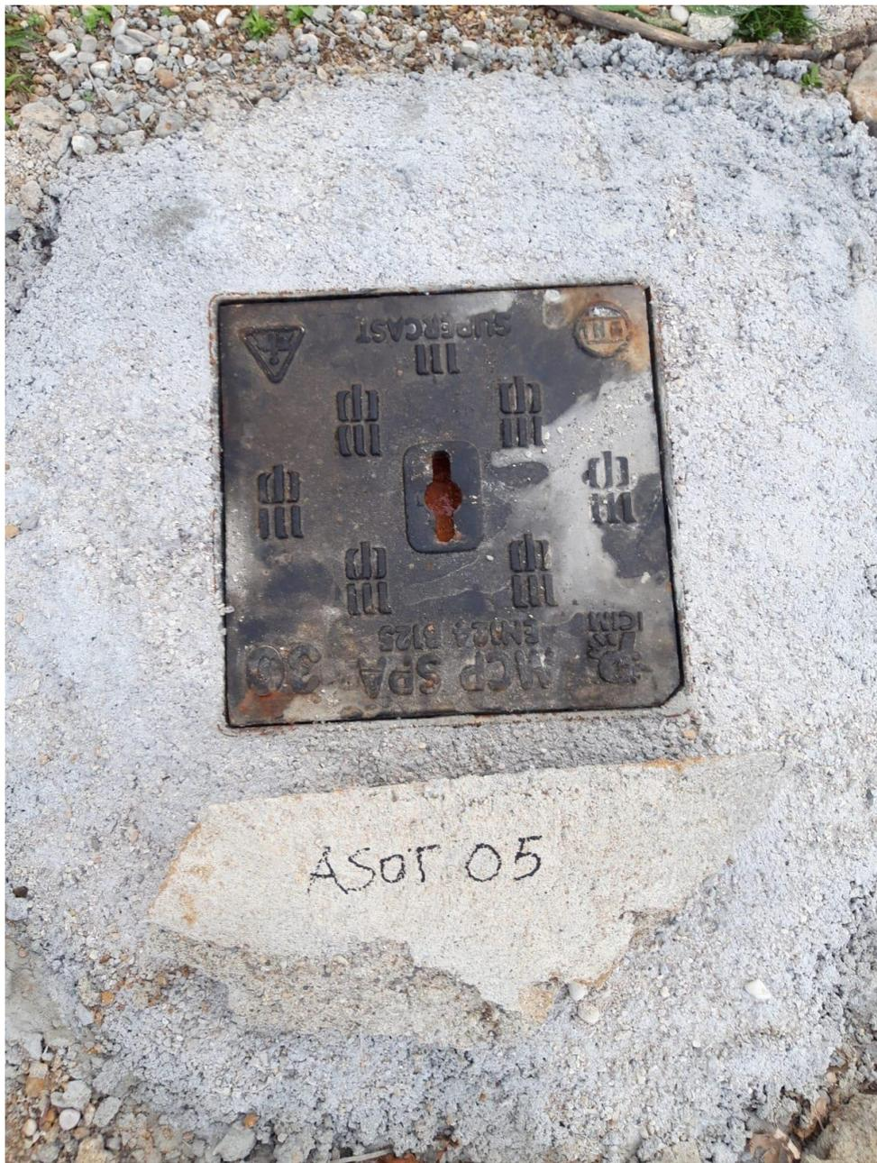
FIGURA N. 17 - Piezometro AST\_05
