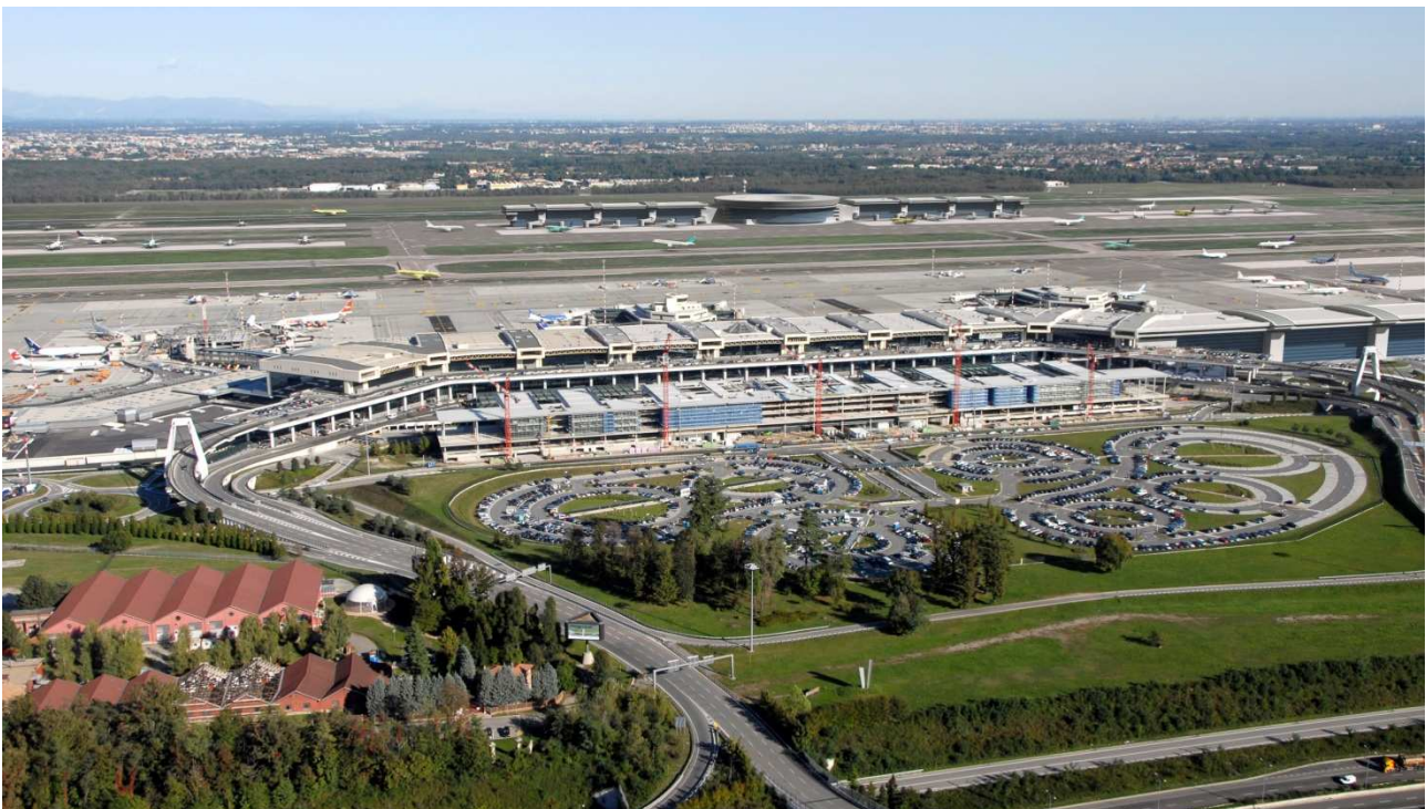
Figura 8-2 Terminal post operam
