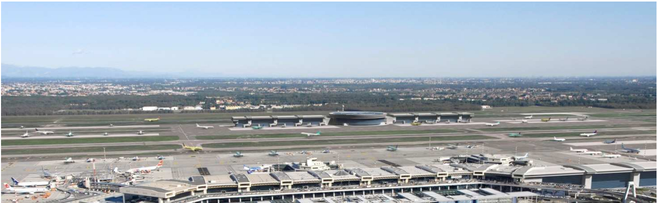
Figura 8-1 Terminal post operam
