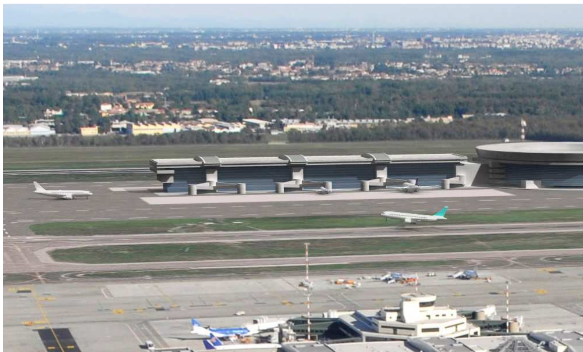
Figura 8-4 Terminal post operam
