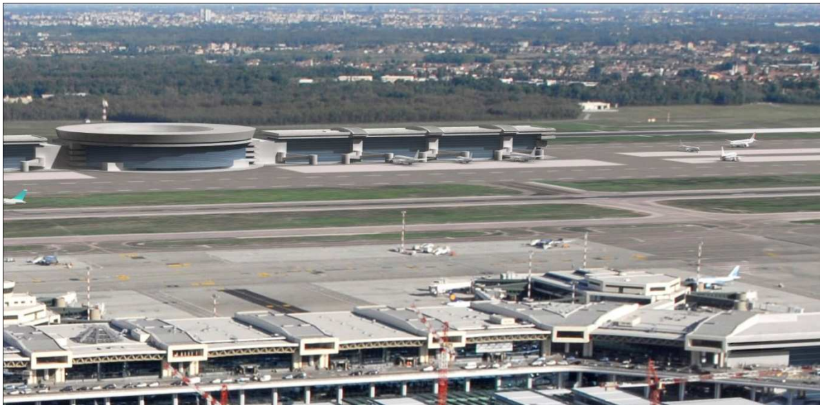
Figura 8-3 Terminal post operam
