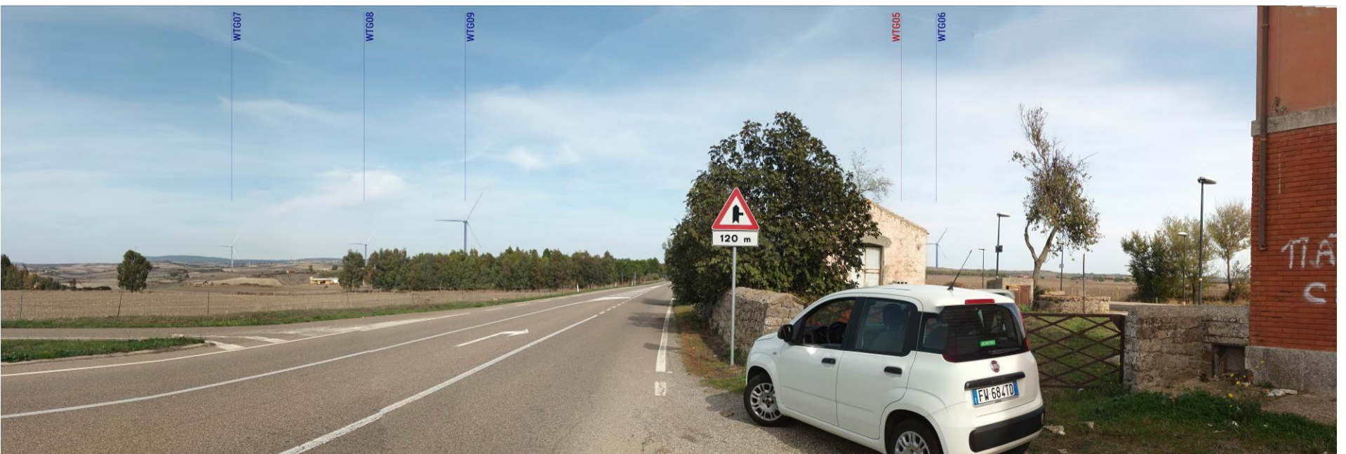
Vista 7b post operam
