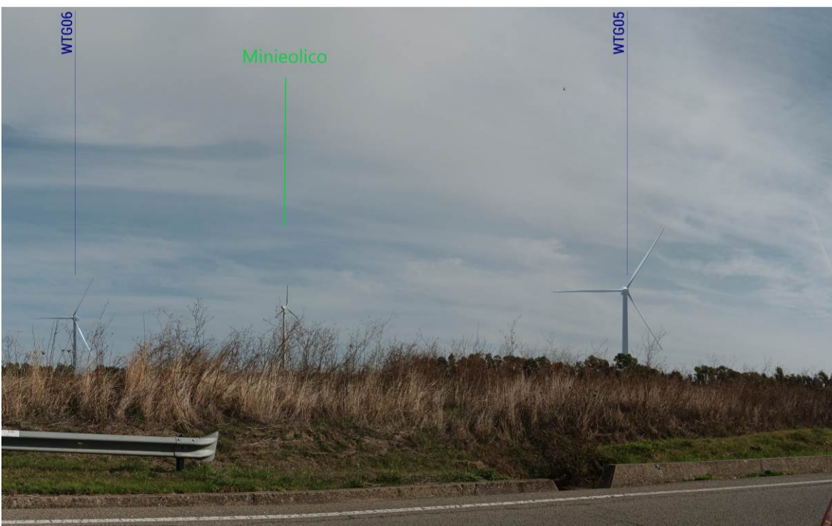
Vista 6b post operam
