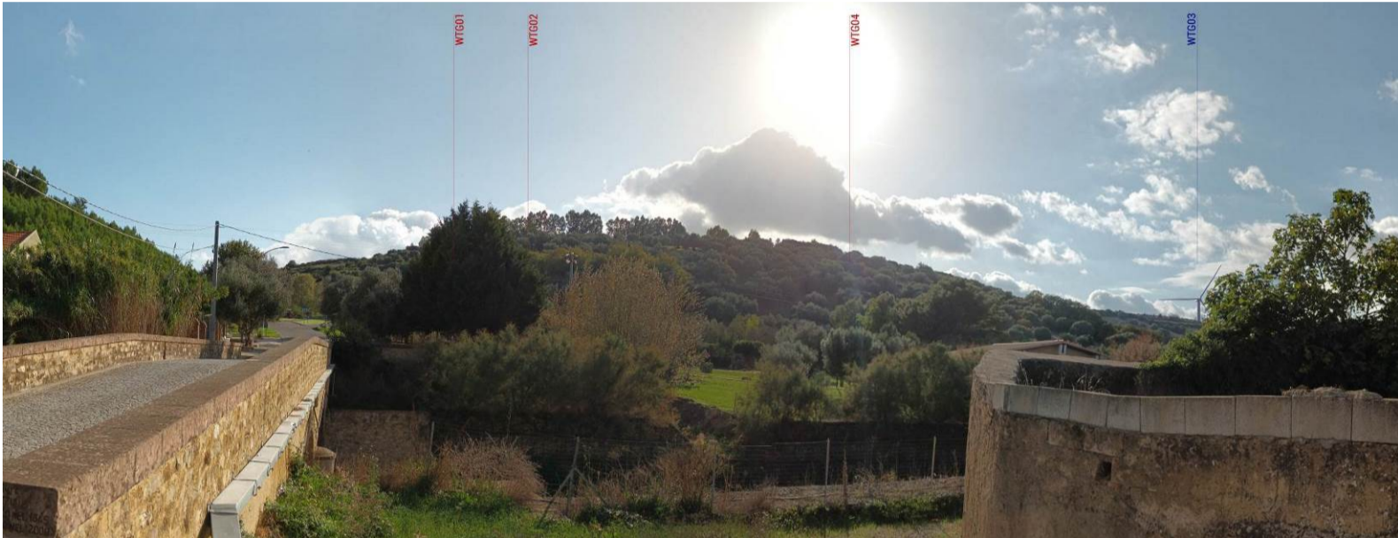
Vista 4_1a post operam
