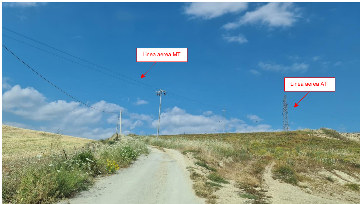
Figura 2.2 Linee aeree AT e MT
