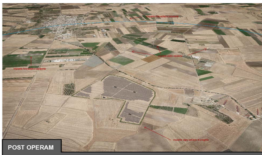
Figura 45 – VISTA 3D 1 POST OPERAM
