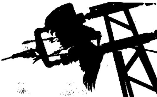
*With its extremely long wings the White Stork has bridged the insulators and was killed by the electric flow through its body.*
