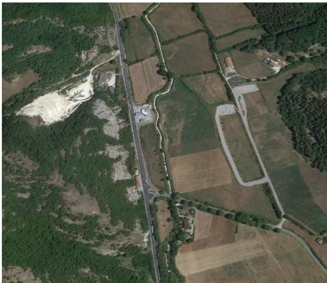
Figura 8.18 – Area cantiere SGR2
