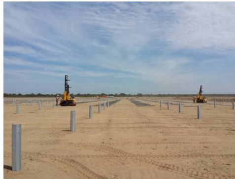
Driving omega piles phase
