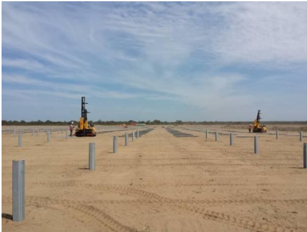
Driving omega piles phase
