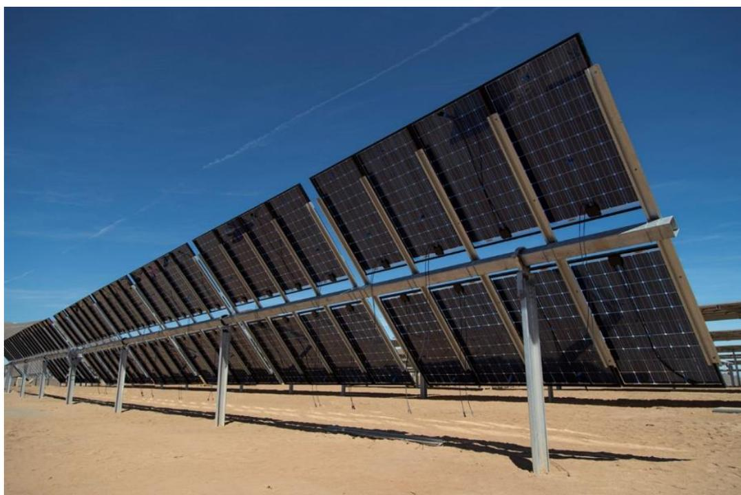
Figura 11 - Particolari struttura di sostegno moduli (<https://soltec.com/soltec-supplies-sf-utility-trackers-for-utility-scale-test-bed-with-bi-facial-pv-modules/>)
