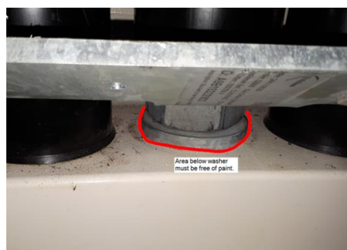
Picture 1: Illustrating paint to be removed on tower flange below the washer.
