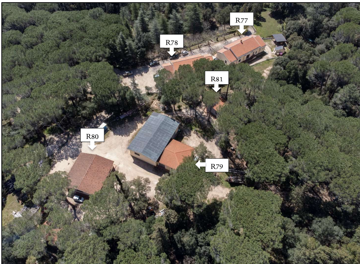
Foto 61a: R77-Buffer 500 m; R78-Buffer 500 m; R79-Buffer 300 m; R80-Buffer 300 m; R81-Buffer 300 m
