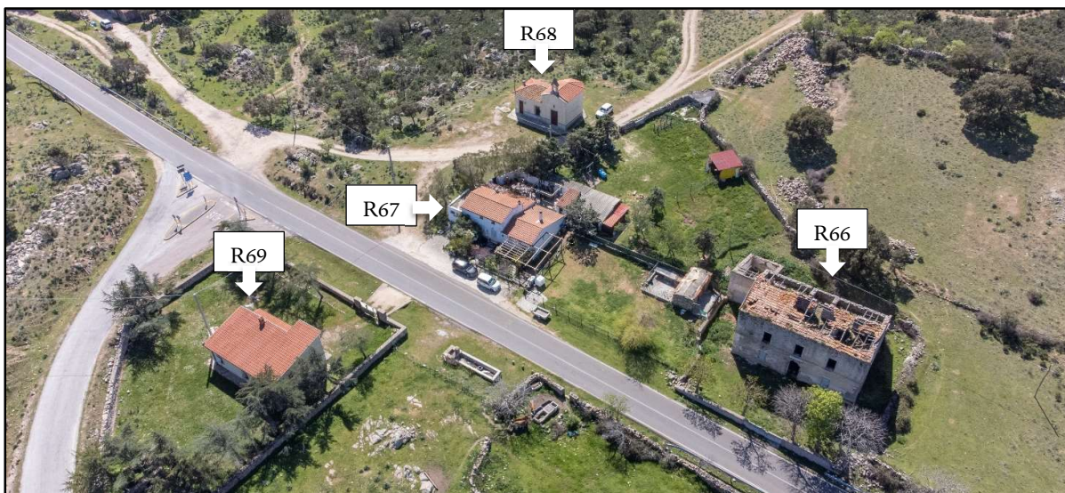
Foto 55b: R66-Buffer 0 m; R67-Buffer 500 m; R68-Buffer 500 m; R69-Buffer 500 m
