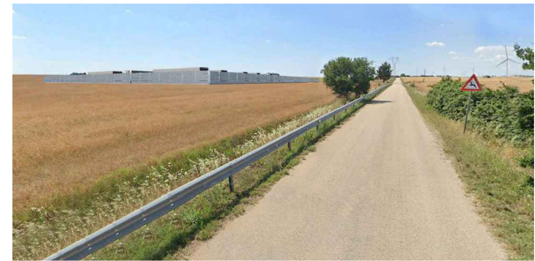
Post operam (in primo piano l'area BESS)
