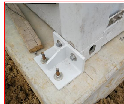
Concrete Foundation: Anchor Bolt Installation
