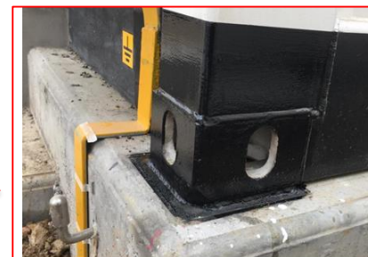
Welding installation: The container bottom frame is welded to the embedded steel plate
