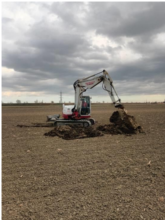
Trial Pit Zona 5
