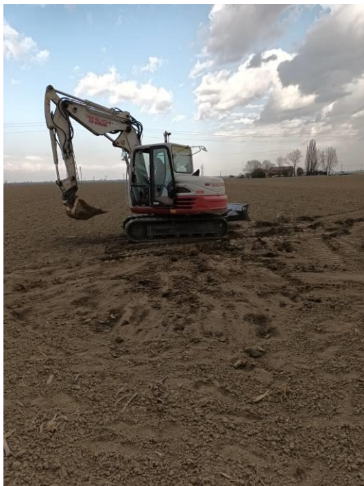
Trial Pit Zona 6
