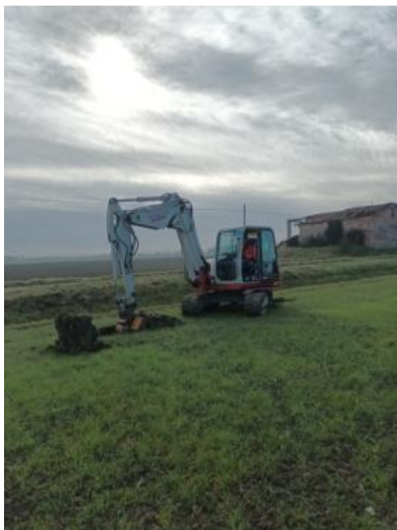
Trial Pit Zona 1
