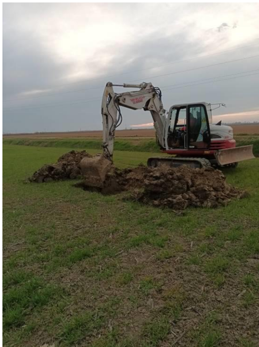
Trial Pit Zona 2
