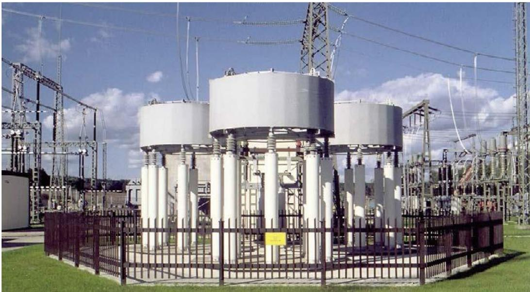
Figura 36 - shunt capacity reactor - fonte Siemens
