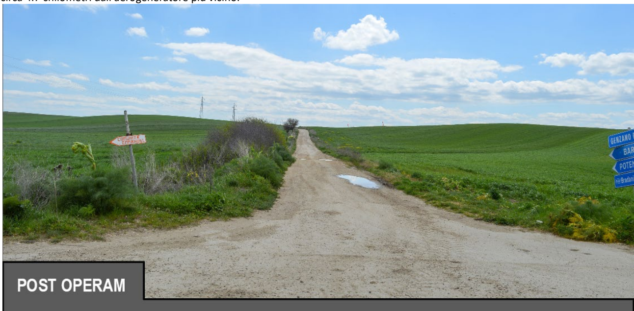
Figura 44 - F3 - POST OPERAM
