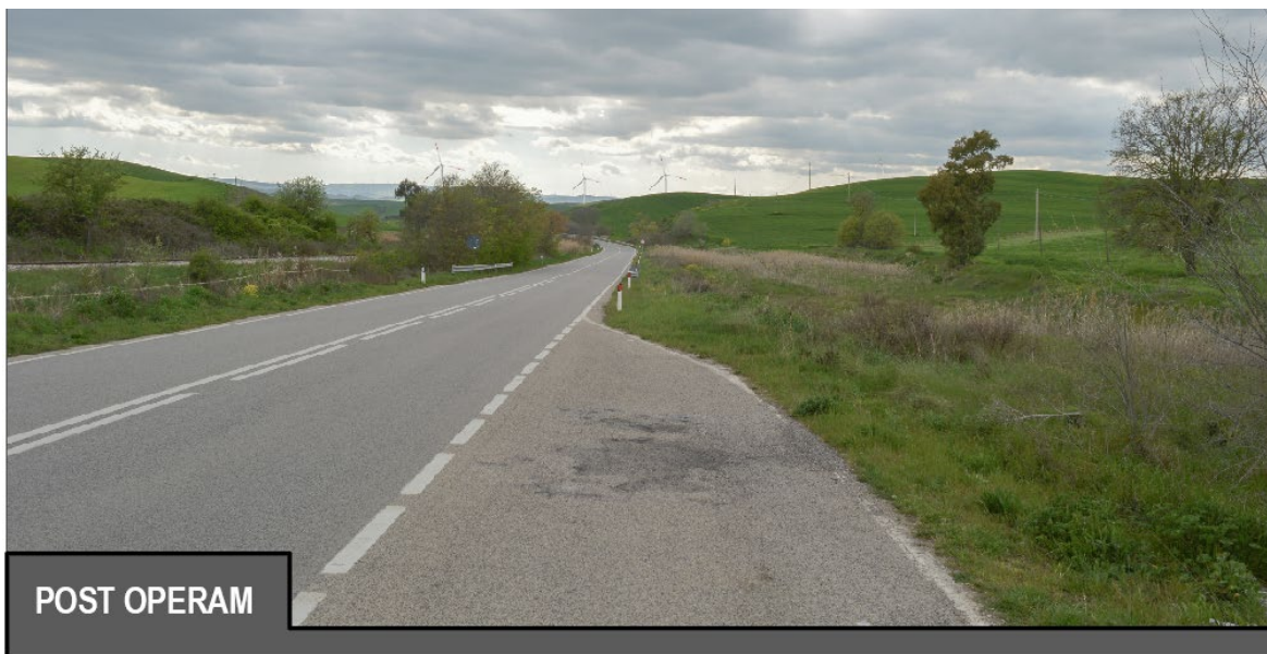
Figura 53 – F7- POST OPERAM
