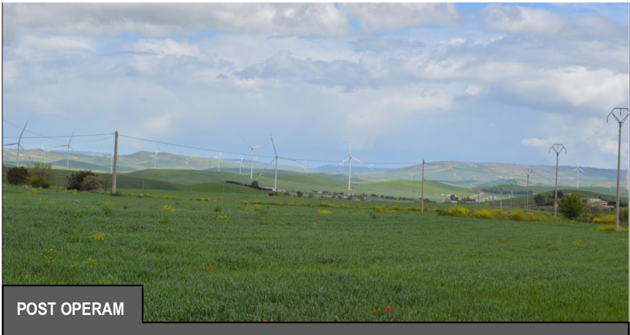
Figura 76 - F19– POST OPERAM
