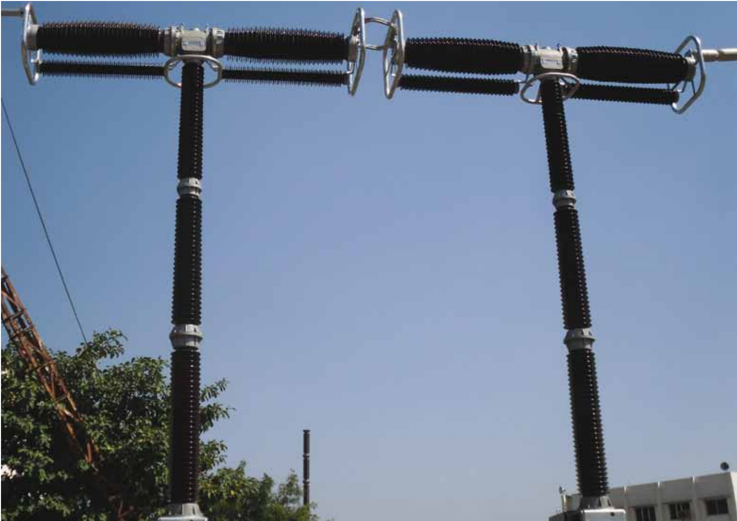
3AP4 FI 800 kV Live-tank circuit-breaker
