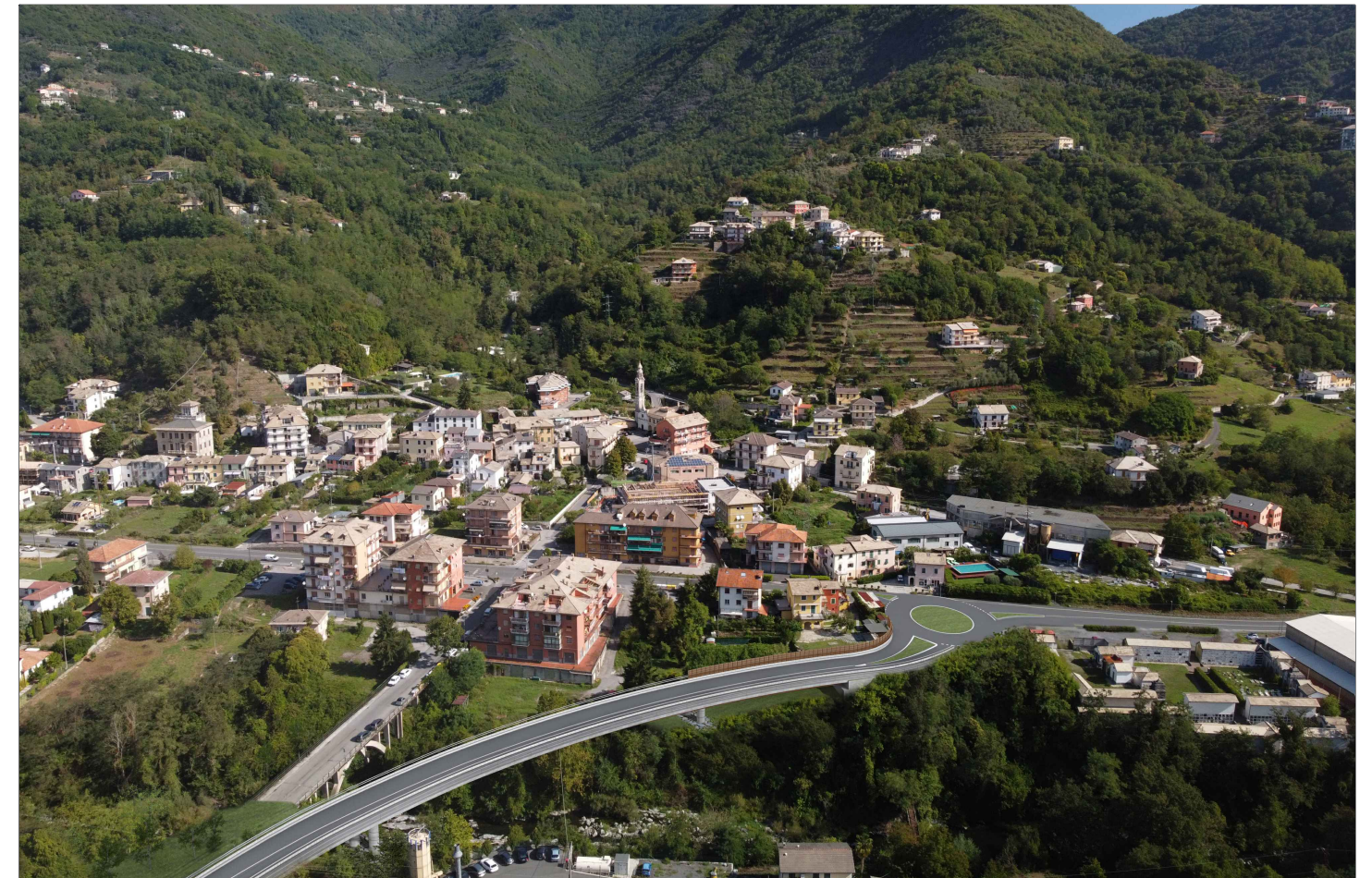
Vista 12 - Post operam
