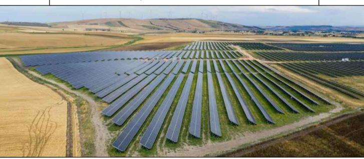
SQUINZANO\_19 PROGETTO DI UN IMPIANTO AGRIVOLTAICO PN<sub>AC</sub> 40 MVA GENERATORE FOTOVOLTAICO PN<sub>DC</sub> 31,56 MW (PN<sub>AC</sub> 26 MVA) + ACCUMULO PN<sub>AC</sub> 14 MVA
