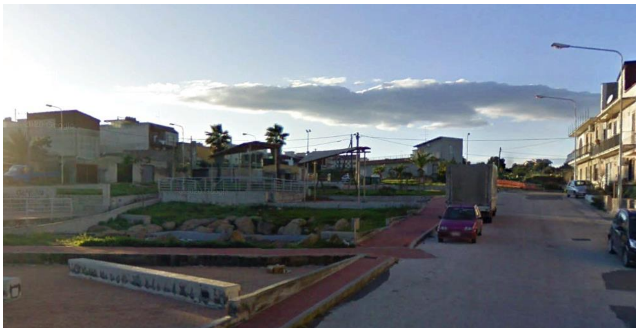
FOTO 22.1 ANTE OPERAM - VILLASMUNDO Via Cavour
